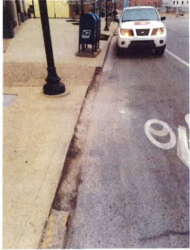
Curblin 100 East Vine St.after
