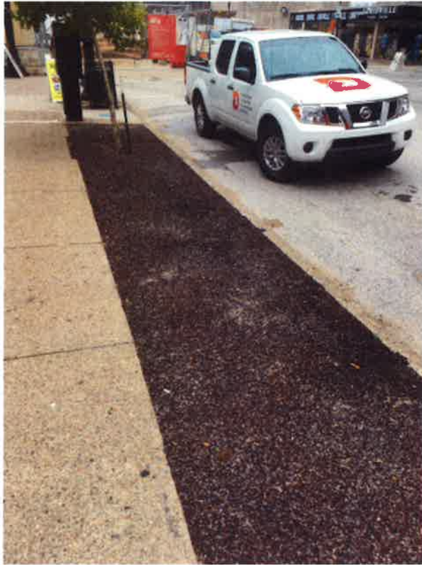
LARGE AREA WITH POROUS PAVE
