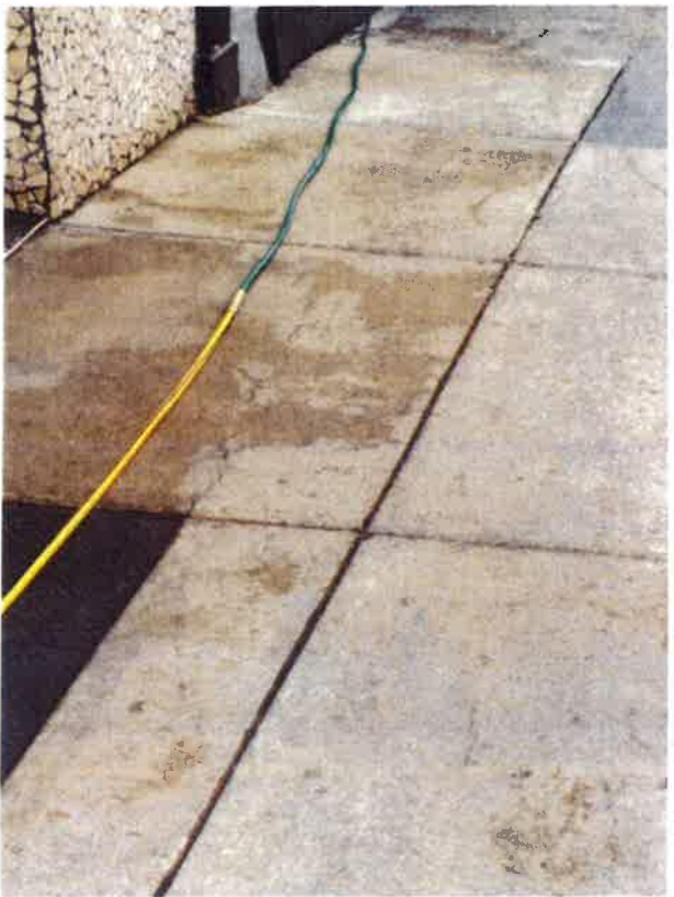
GUM REMOVAL USING HOT WATER PRESSURE WASHER
